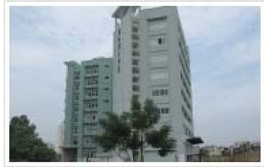
Main building of IOP
