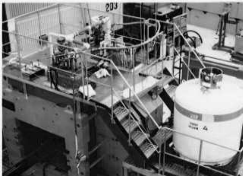
Installed with return yoke at KEK
