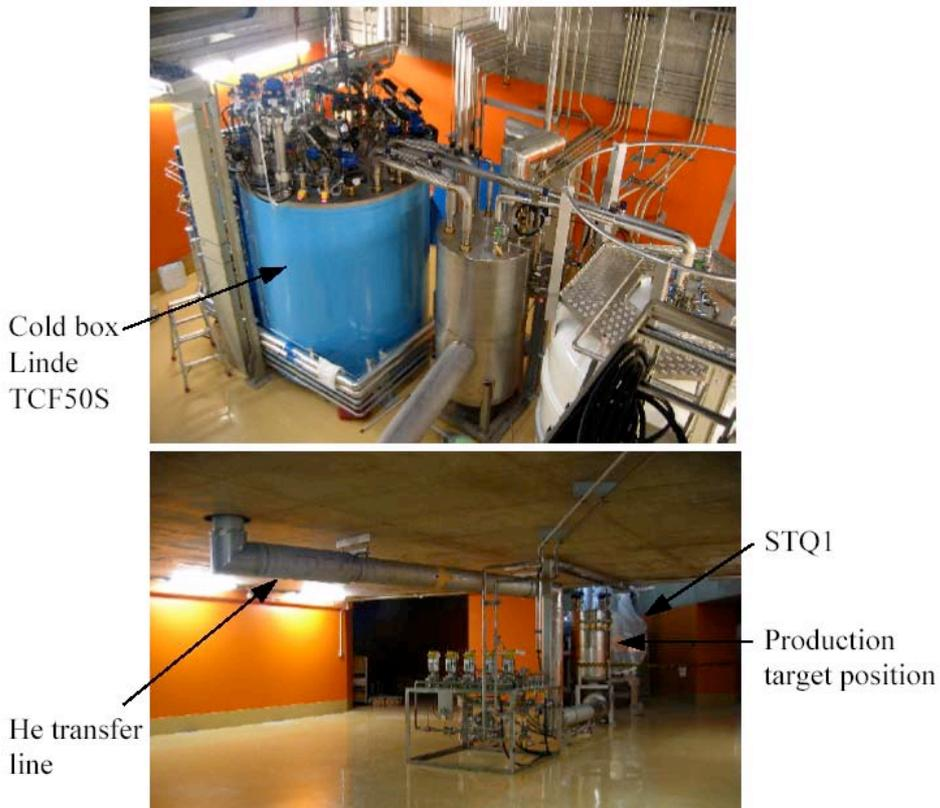
Fig. 4-b. Photographs of the cryogenic system for the first-stage quadrupoles.
