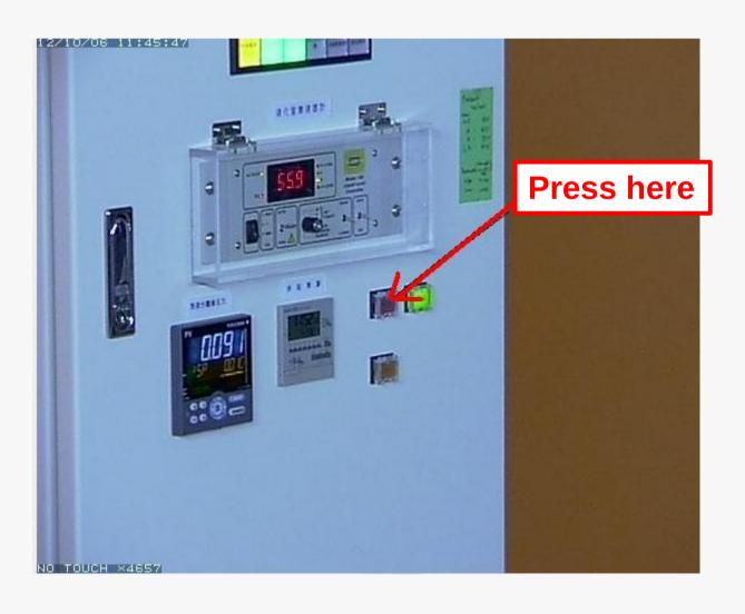
To start the filling of tank manually, first switch ① from "自動" to " $\lambda$ ", then press ② (起動)
