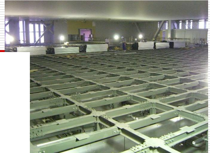
Making a double floor
